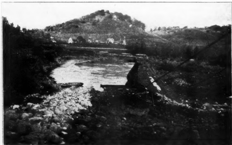
Gettings the Pit Opened; a View Shortly After Start
